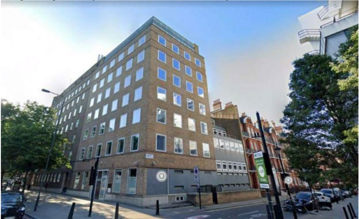
Existing Building from Marylebone Road, and from across Marylebone Road
